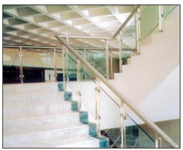
Stainless steel handrails in combination withy acrylic balusters and glass guardrails. The stainless steel clamps were specially designed to weld the top rail to the balusters and the baluster to the base plate at each step. The clamps are forged and machined to perfection and are designed as a two-piece system whereby the glass can be replaced without removing the clamps from the balusters.
